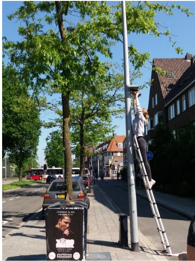
Figure 38: Mounting the cameras on the lamp post.
