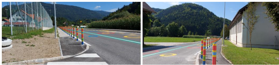
Fig. 9. Case in which traffic bollards obstruct the view from the side road.
