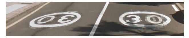
In this way, the driver's attention is drawn in a positive way, to the speed limit that he must respect, especially when he is overtaking, driving in the left lane and in the right lane there is a higher vehicle and he cannot see the vertical sign, vegetation, or the sun prevent him from seeing the speed limit sign.
