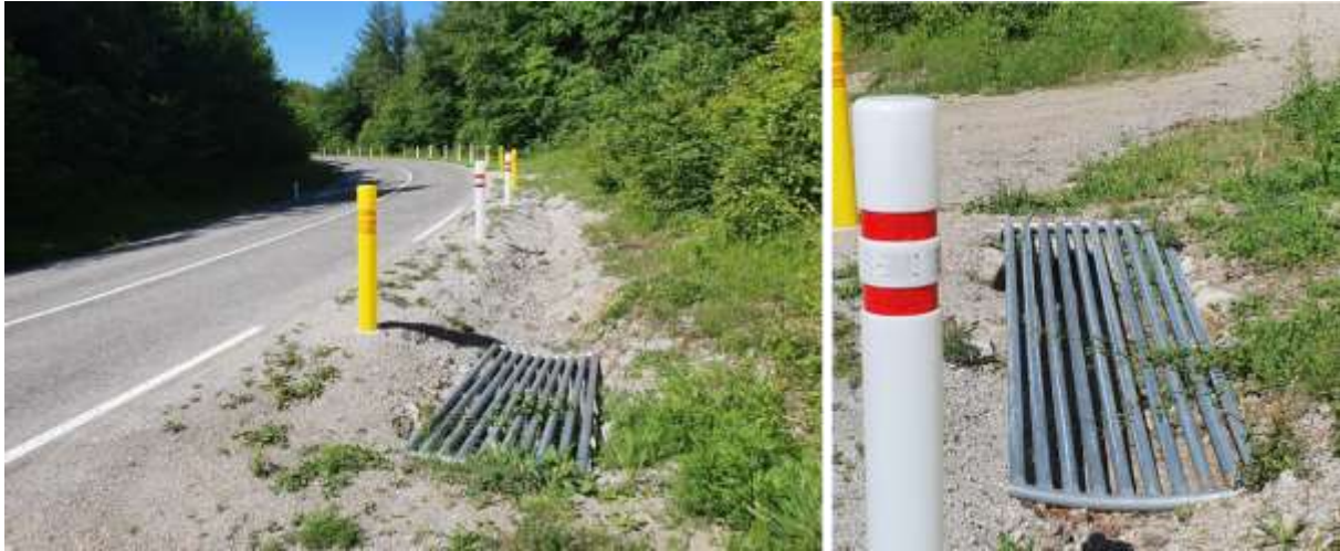
Figure 5 – Iron grid covering the road ditch culvert.
