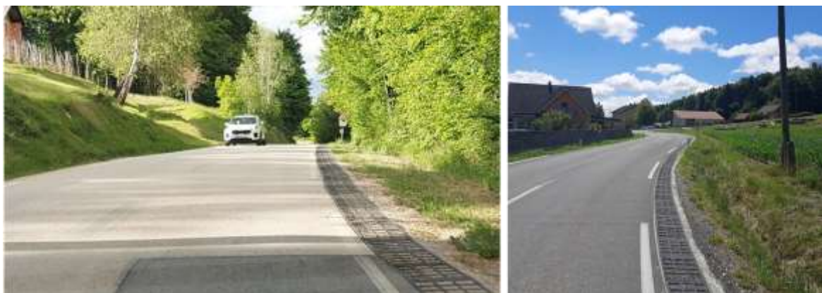
Figure 9 – Trapezoidal mesh panels in the road bank.
