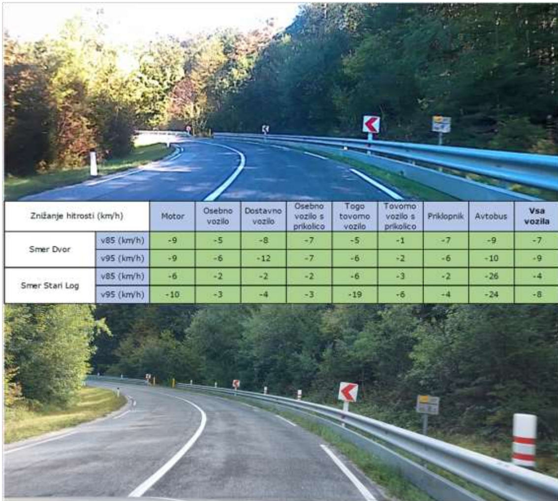
Figure 4 – Results before/after hidden speed measurements on one curve that needed to be upgraded after H.F. evaluation.
