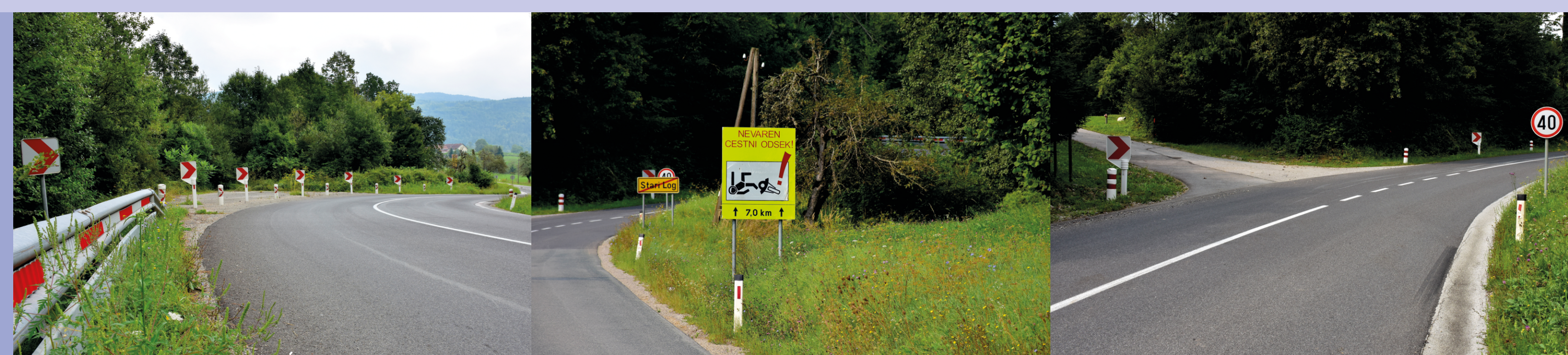
Adding red/white elements in the groove of the road safety barrier.
