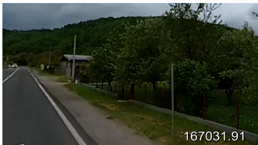
Figure 2 – Pillar on chainage Km~167+040 with a missing traffic sign
