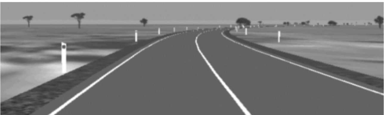
Figure 2.17: Edge line marking with reflector guide posts
