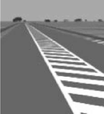
Figure 2.16: Hatched centre line treatment
