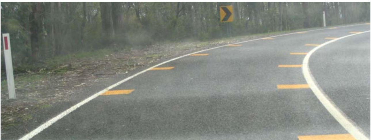
Figure 2.19: Peripheral transverse line markings and guide posts
