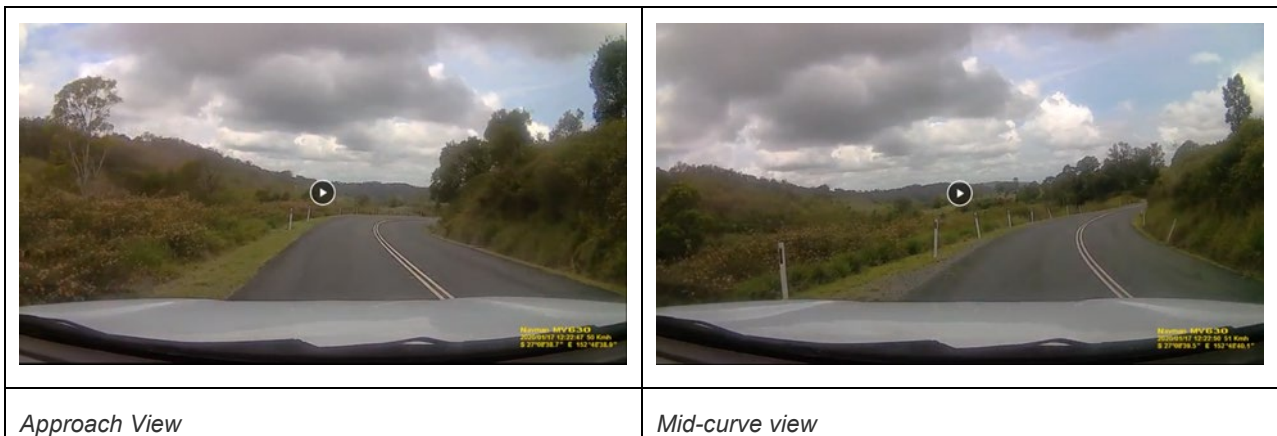
Figure C.16: Views of the approach and mid curve for Curve B at Site 5 (southbound direction)
