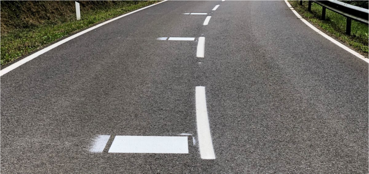
Figure 2.8: Peripheral line marking installed to increase lane separation in Luxembourg
