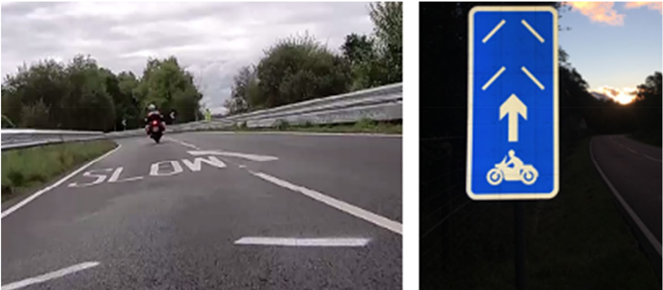
Figure 2.25: Gating-type line marking treatment trialled in Scotland
