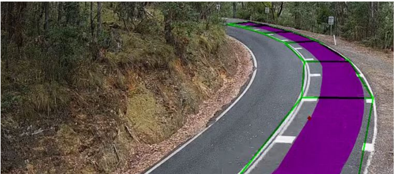
Figure 2.24: Peripheral line marking treatment trialled in Victoria
