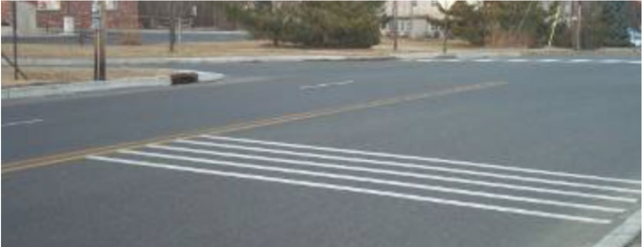
Figure 2.3: Example of typical application of rumble strips
