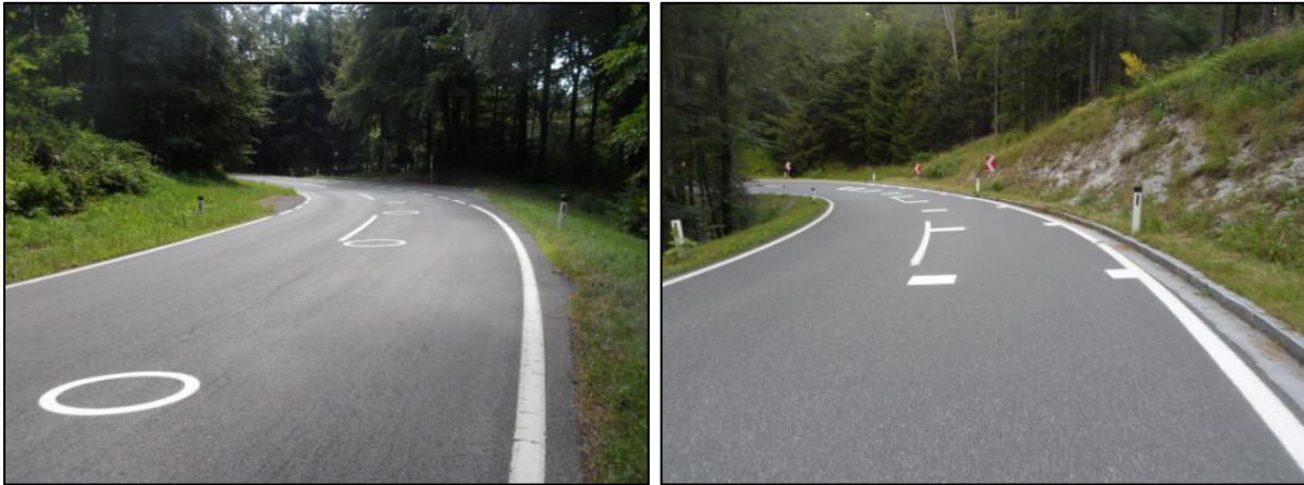
Figure 8 Shape of road markings; A: elliptic design, B: psychological brake (bar design)
